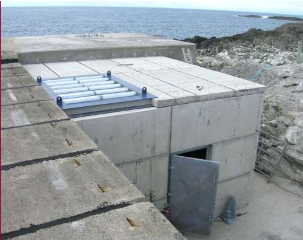
Turbine hall & acoustic attenuator
