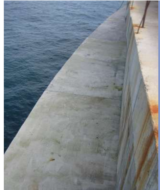
Mutriku new outer wall
